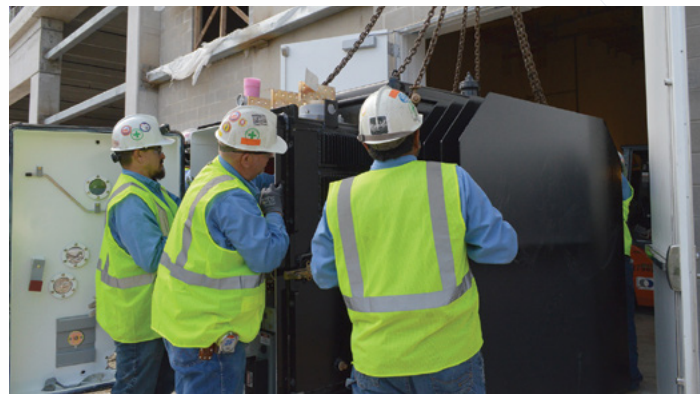
An Integrated Underground Construction & Maintenance Crew working safely.
