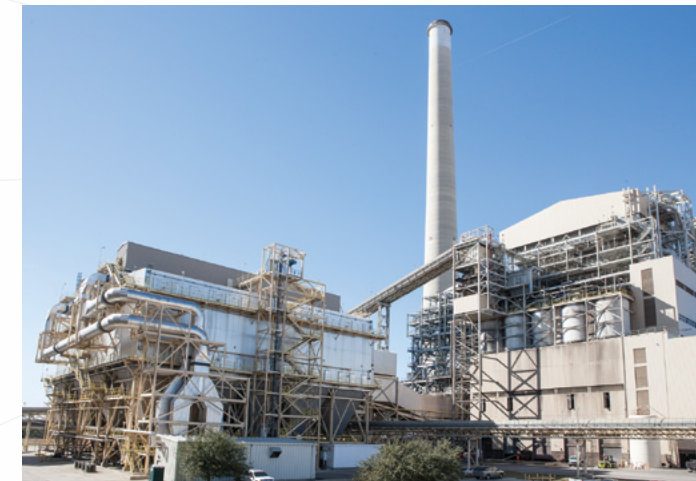
Nearly 70 CPS Energy employees received skills training to transition into other positions at CPS Energy. Everyone who worked at Deely still works for CPS Energy in another capacity.
